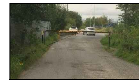
Current access control is a manual swing gate. When shut users are expected to walk around the post which is approximately 0.8m wide with a small embankment to the side.
